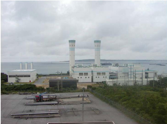
Miyako No.2 Power Station
