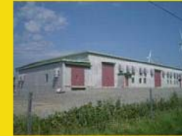
Wind Power Stabilizing demonstration (Tomamae)
