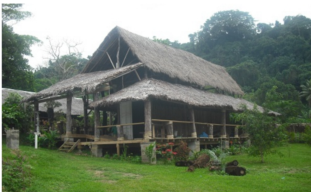
Figure 7 : ACTIV training Centre outside Port Vila, Vanuatu
