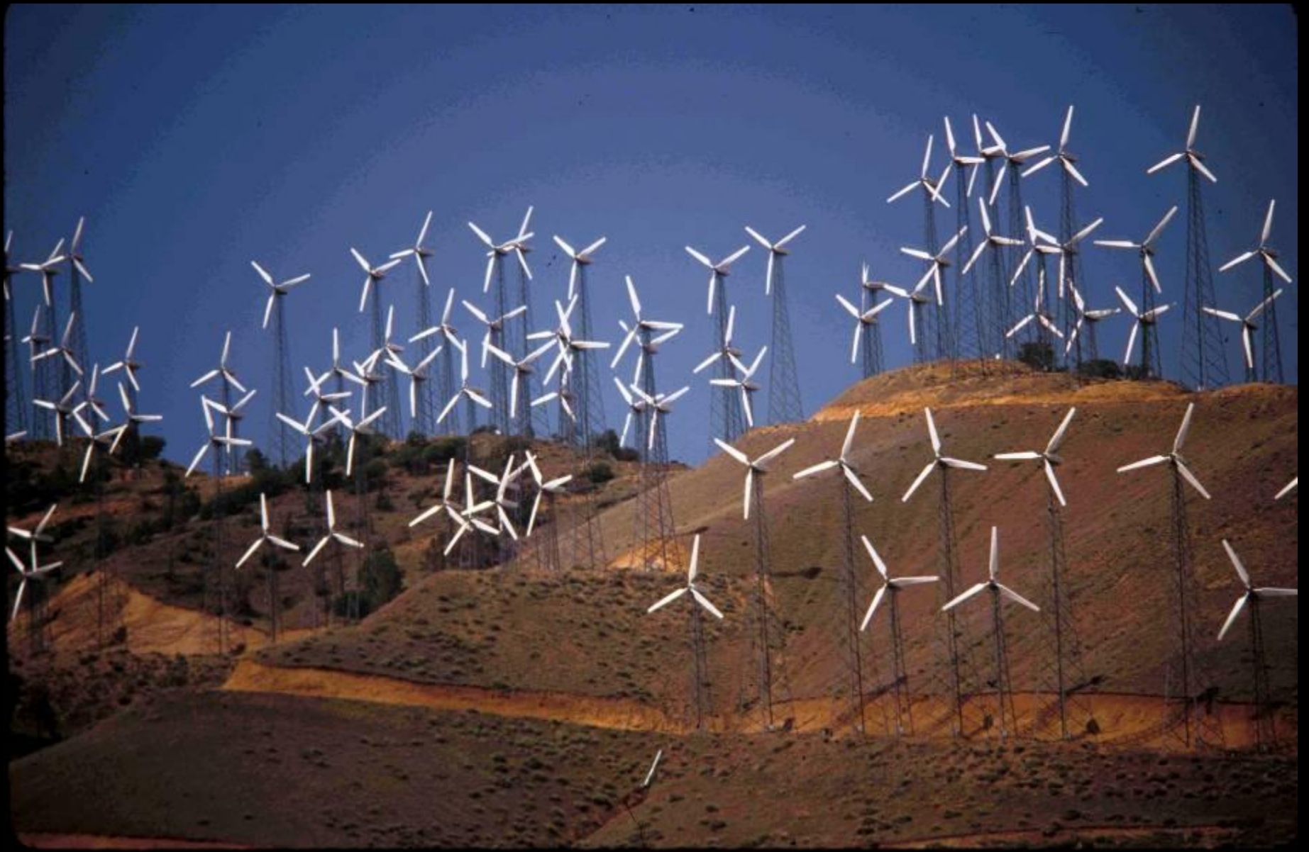
Tehachapi Pass, California
