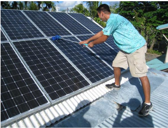
Final cleaning of the panels
