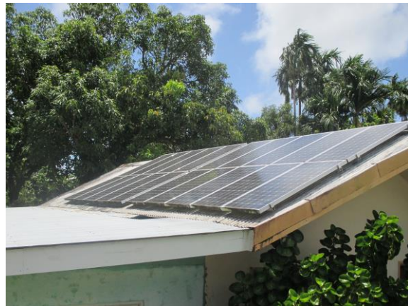
Completed panel installation
