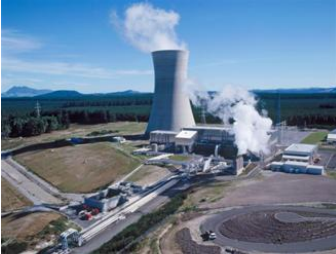
Ohaaki Geothermal power station
