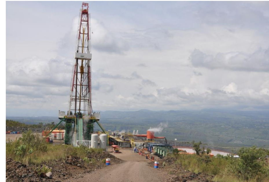
A drilling rig at Menengai, Kenya (source: Kenya GDC)
