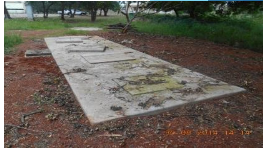
Anaerobic Baffled Reactor (ABR)
