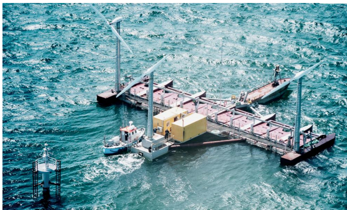
Floating Power Plant
