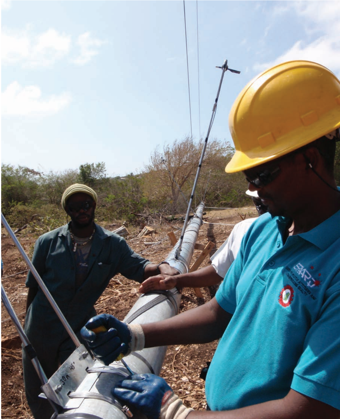
Setting up wind masts in Carriacou, Grenada Courtesy of GRENLEC
