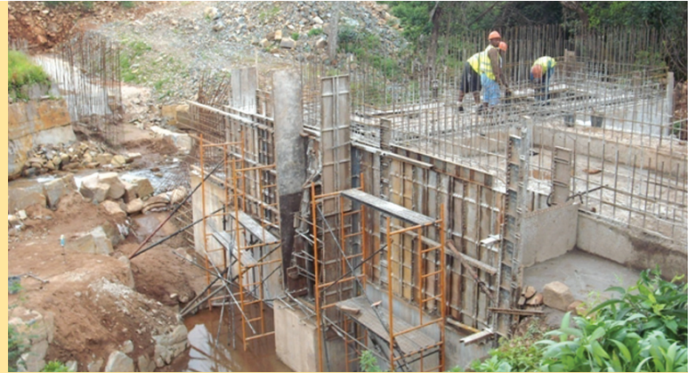
Rotanda hydropower project in Mozambique Courtesy of FUNAE, Fundo de Energia
