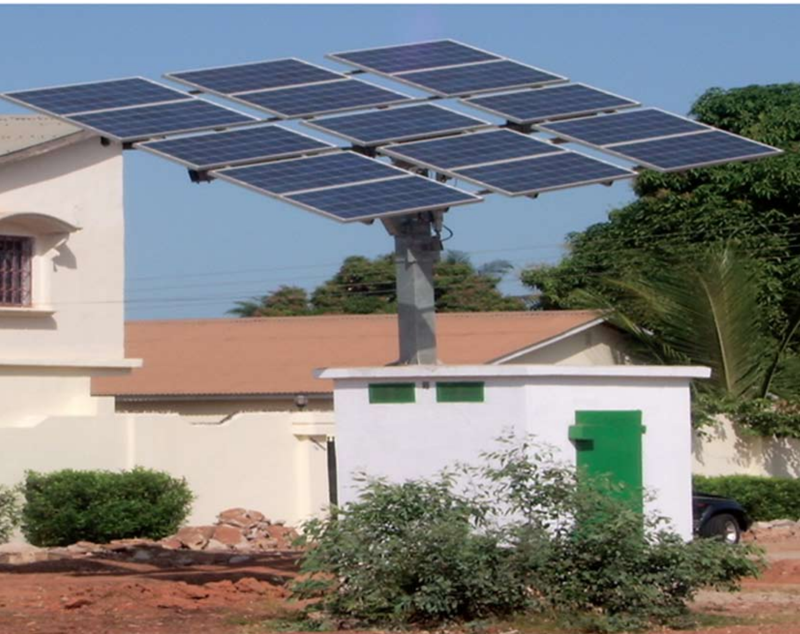
Source: Ministry of Energy, The Gambia
