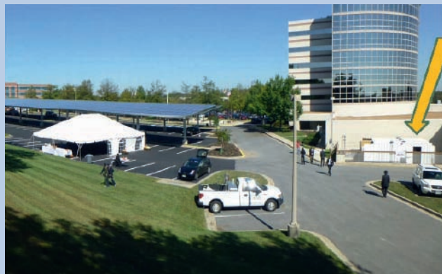
Location of the battery storage site. Source: Cook, C. (2013)
