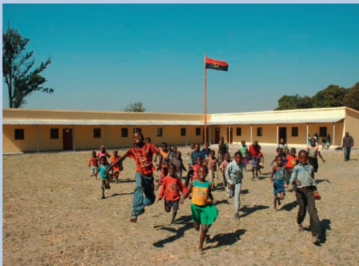
AllCell off-grid solar and battery storage at a school in Angola.
