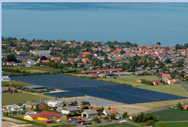
Figure 4: Marstal Solar District heating plant (33 360 m 2 ), Denmark
