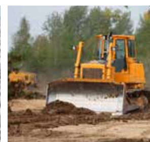
Clearing the site
