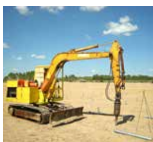
Site preparation and civil works
