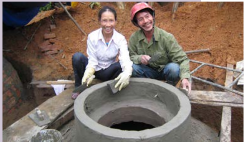
Biogas digester construction in Viet Nam
