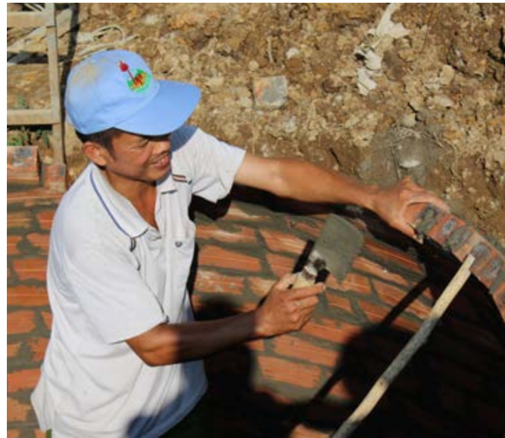
Biogas digester construction in Viet Nam
