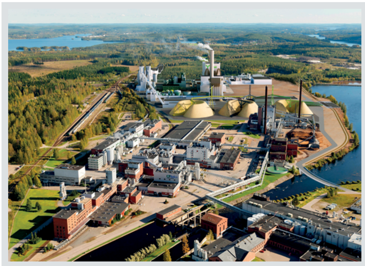
Figure 8 Äänekoski bioproduct mill shown behind the existing plant
