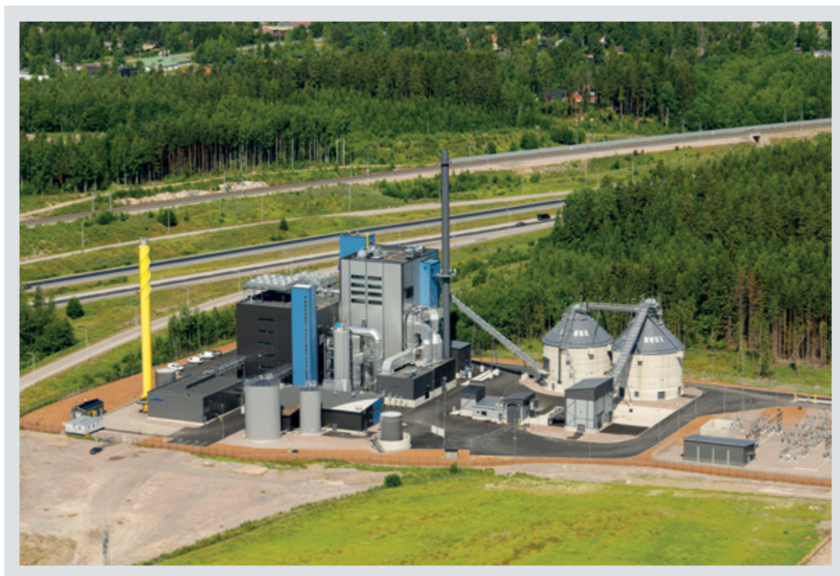
Figure 12 Aerial view of Järvenpää multifuel CHP plant
