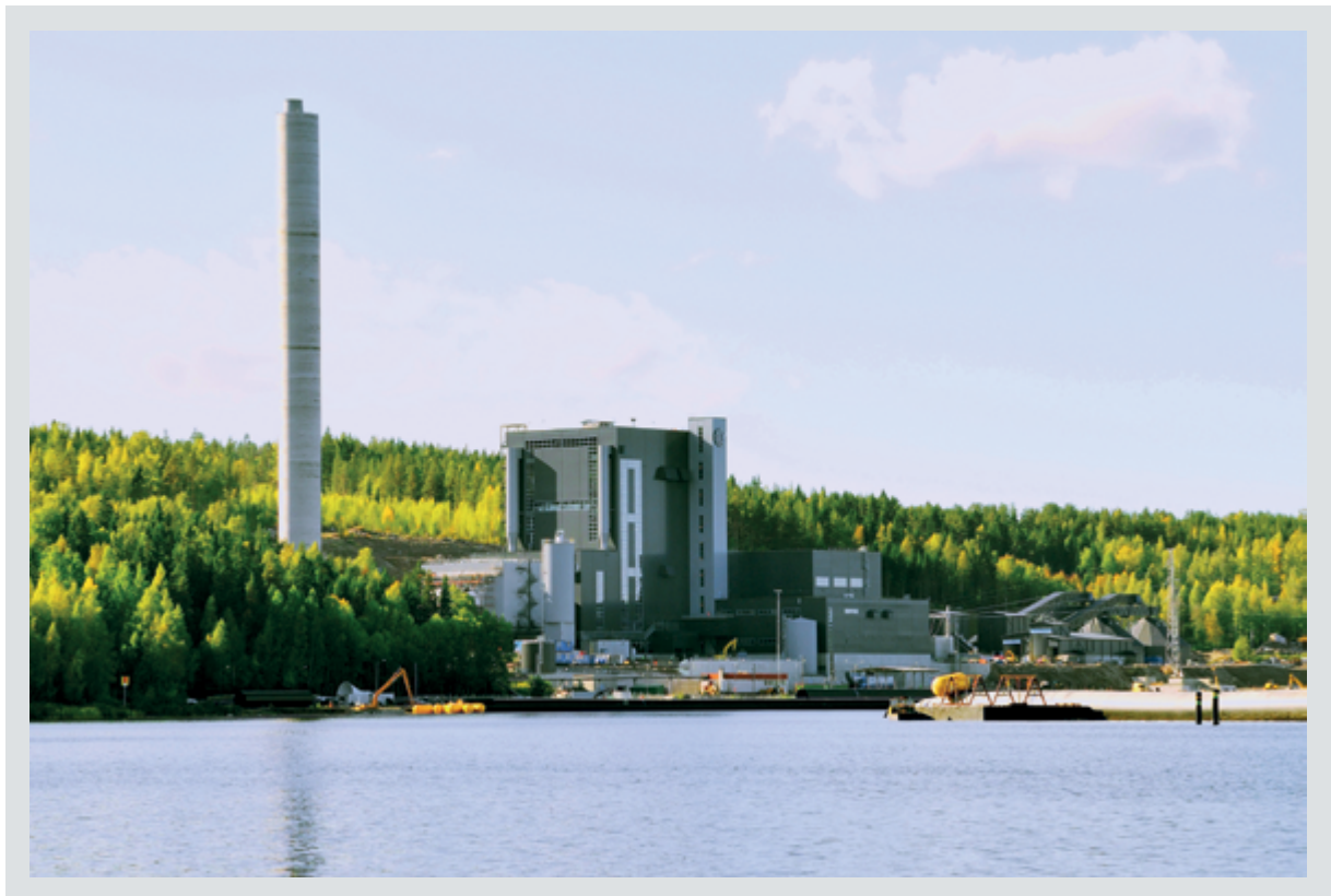
Figure 5 Keljonlahti CHP Plant in Jyväskylä
