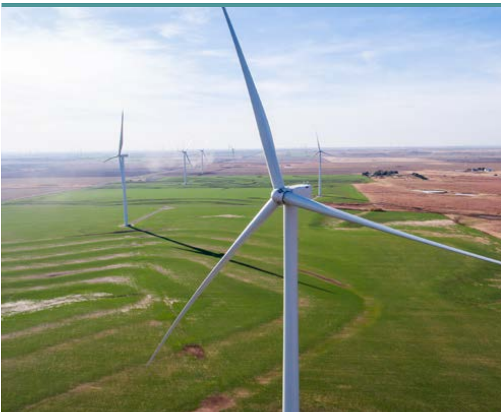
298 MW Thunder Ranch wind project by Enel Green Power of which Anheuser-Busch purchases a portion of the generated electricity through a corporate PPA.
