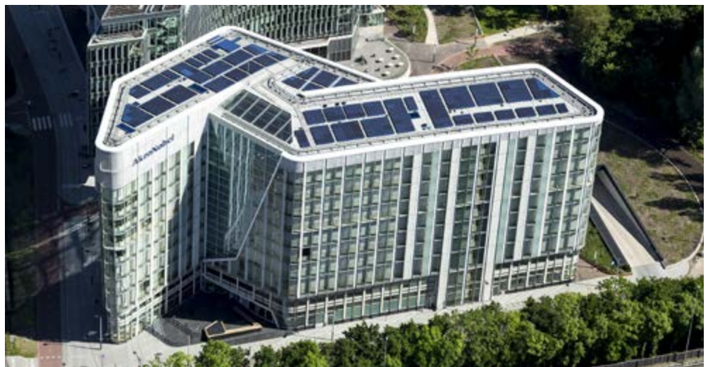
On-site solar PV system at Akzo Nobel headquarters in Amsterdam, Netherlands. Source: Akzo Nobel
