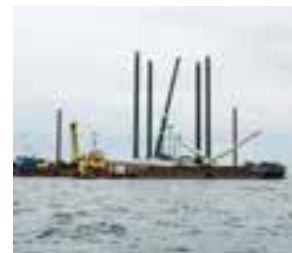
Clearing the site
