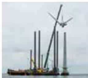
Dismantling the project
