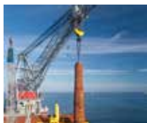
Site preparation and civil works
