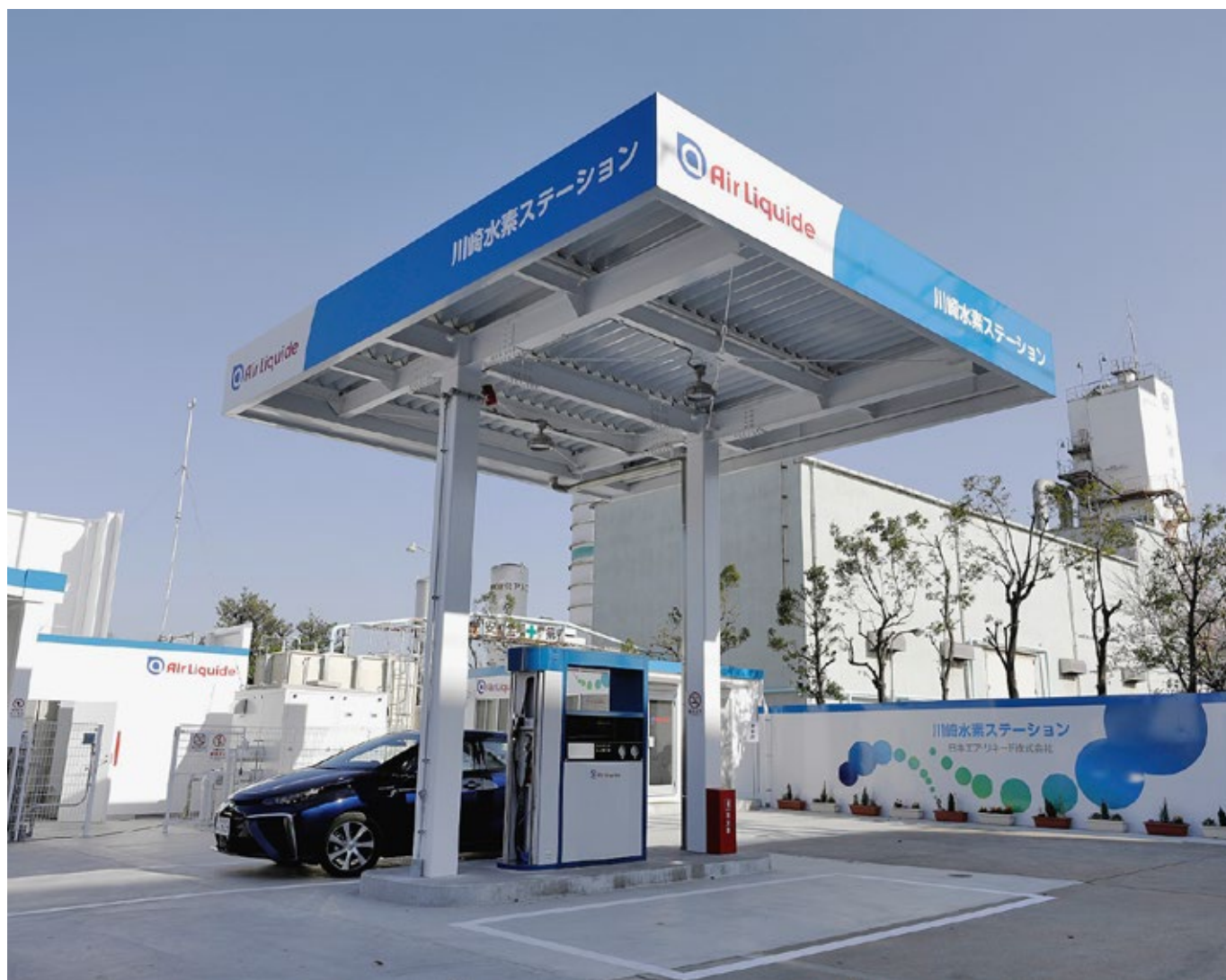
Figure 24: Hydrogen refuelling station in Kawasaki, Kanagawa Prefecture, Japan
