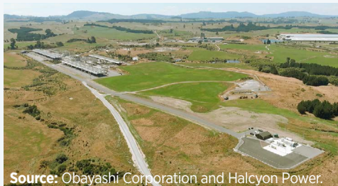
Photograph 5 Demonstration plant for green hydrogen production powered by geothermal energy at the Mokai geothermal field, Taupo, New Zealand
