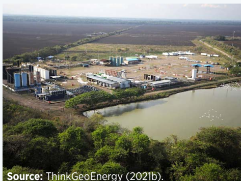
Photograph 3 Geothermal site of the Las Maracas project in Colombia
