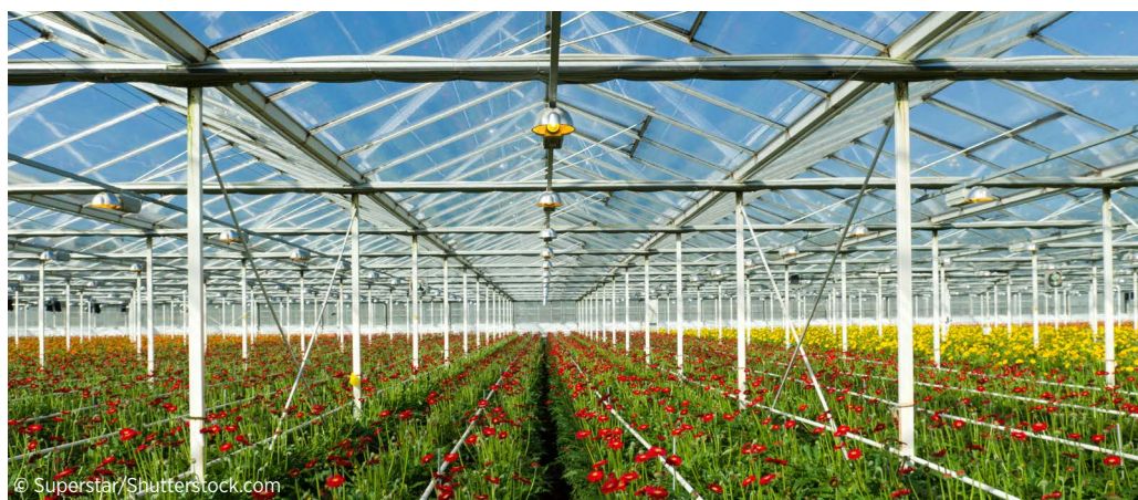
Commercial greenhouse powered by geothermal.
