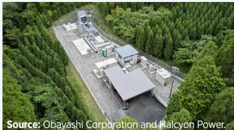
Photograph 6 Demonstration plant for green hydrogen production powered by geothermal energy in Kyushu, Japan
