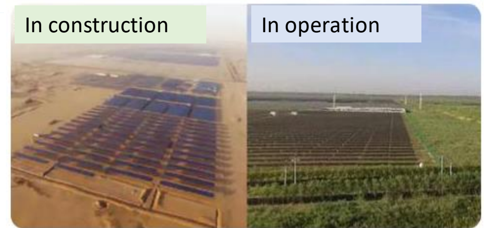
Inner Mongolia PV sand control project
