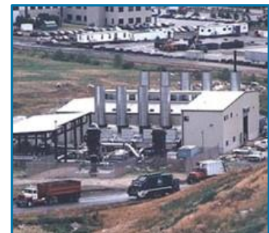
Municipal solid waste incinerator, China
