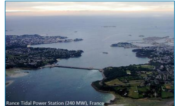
Rance Tidal Power Station (240 MW), France
